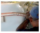
The track can be fixed with blind rivets or self drilling screws in stainless steel A4 (316).
